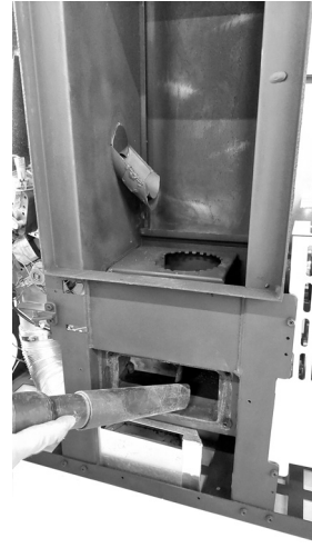
Fig. 59 - Vacuum out the ash
