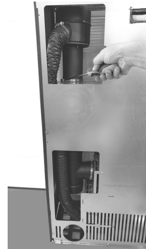
Fig. 36 - Block with clamp
