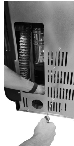
Fig. 38 - Connect the flexible hose
