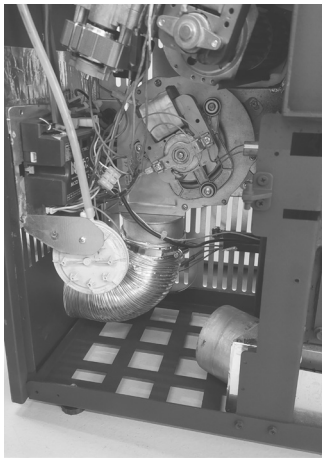
Fig. 30 - Install the pipe
