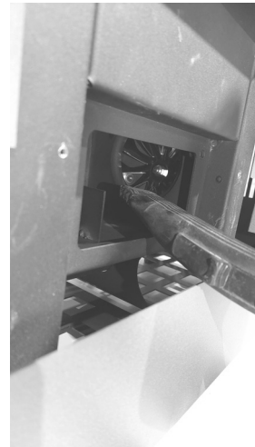
Fig. 61 - Vacuum out the ash
